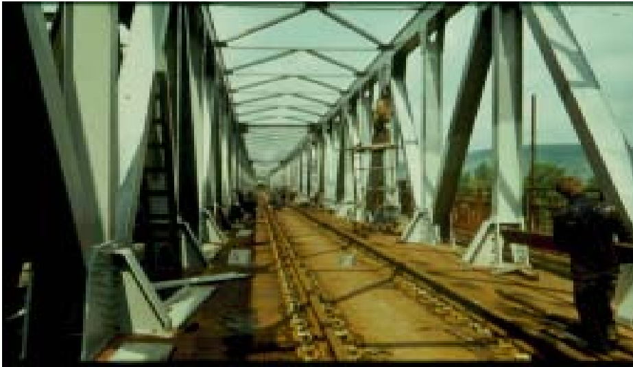
Figure 3. Orthotropic steel-plate floor
