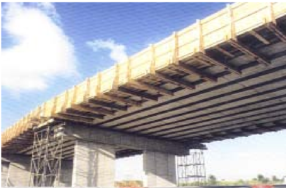
Figure 4. Composite encased beams
