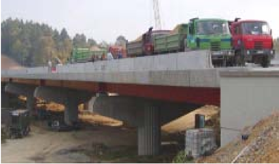
Figure 2. Composite steel and concrete bridge structure
